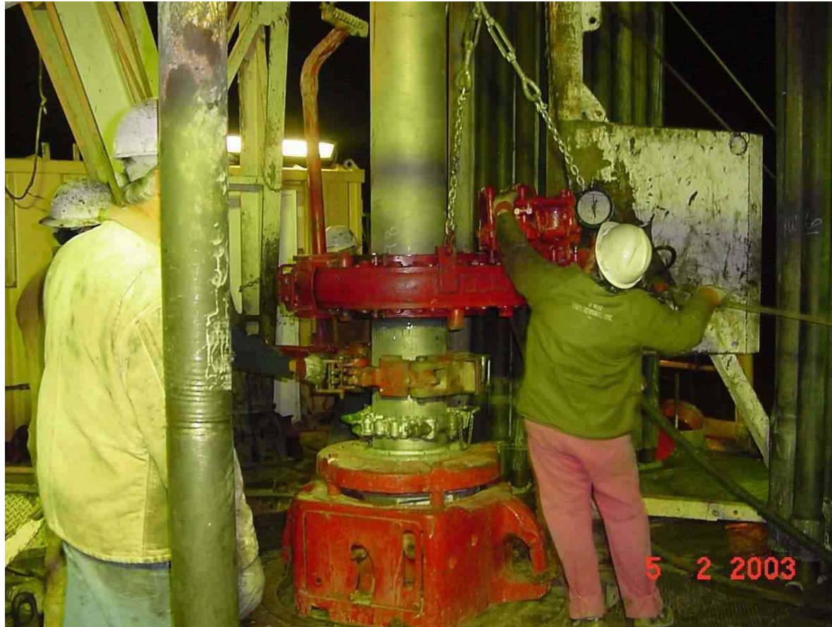
Running in the well with 16" Titanium casing In geothermal well
