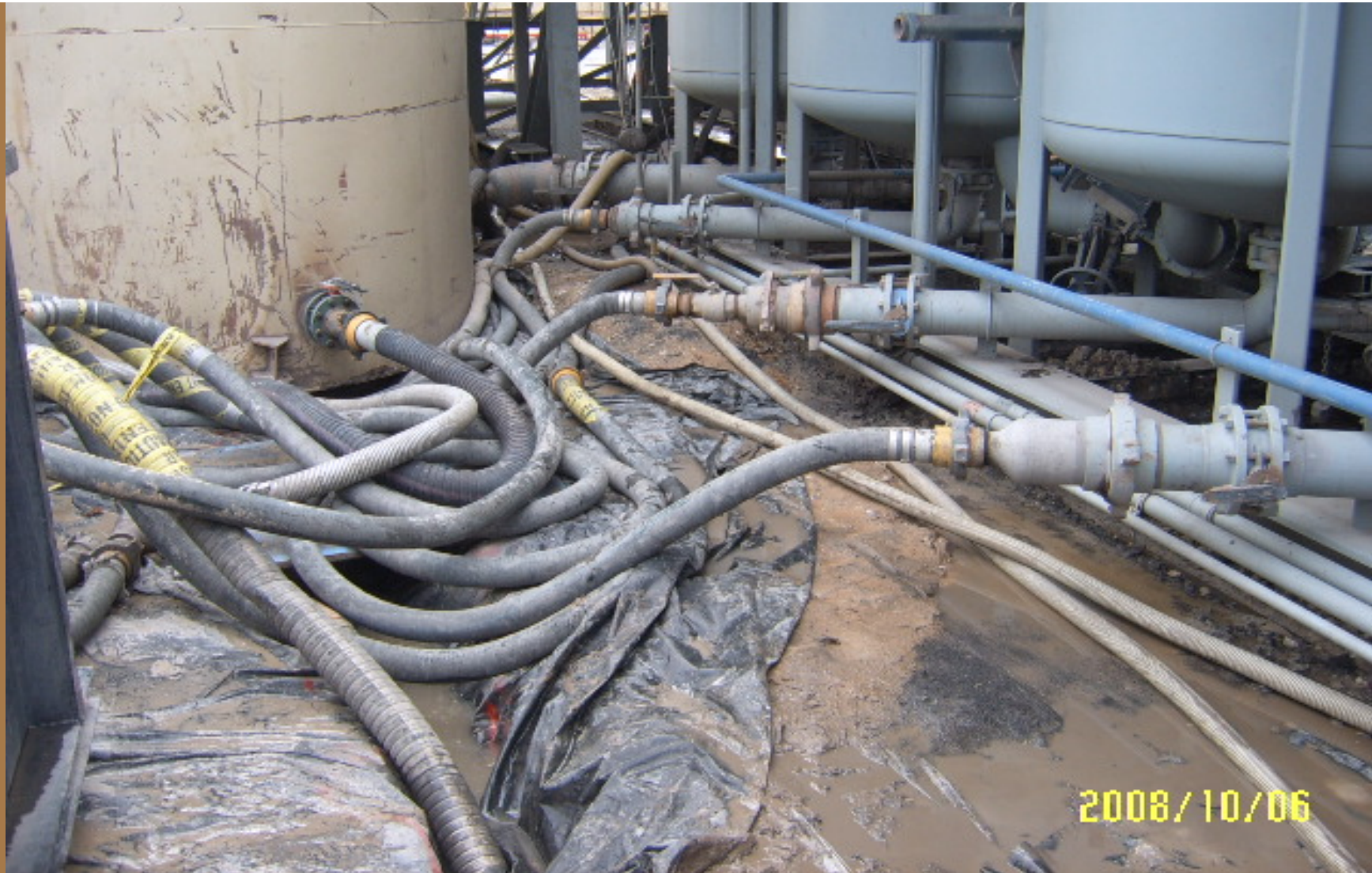
Figure 3: Field Rig-up of LCM Recovery Tank
