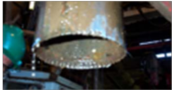
Fig. 11. A chemical cut of 5 1/2-in. casing.
