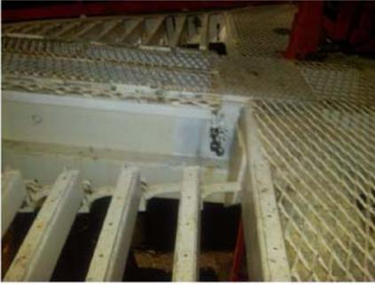
Fig. 5 – Welded Diving Board Design and Collision Damage
