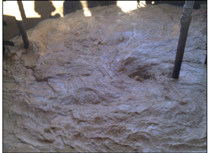
Figure 10: MCP mixed inside the tank and agitated using the gun lines.
