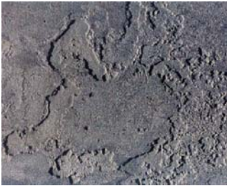
Figure 9 Stress Related Cracking
