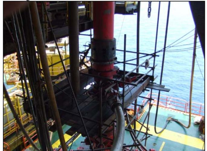
Figure 20. Picture showing the HOLD 2500 Rotating Control Device installed in the riser above the stack.
