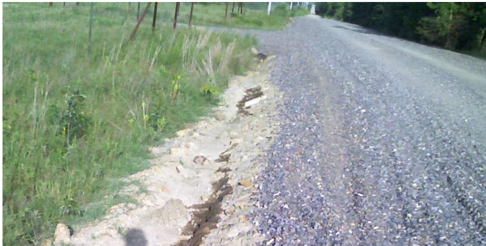
Diesel runoff in roadside ditch on a county road. Oil-based cuttings had previously been roadspread on this road.
