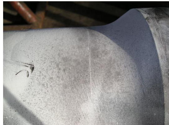
Severe crack found during routine inspections
