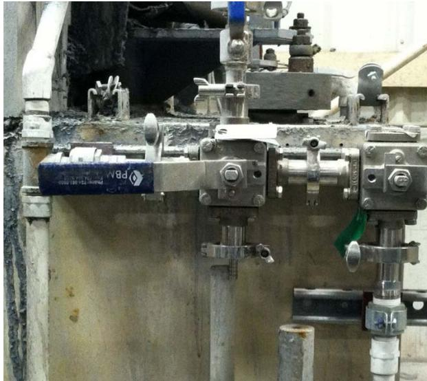
**Figure 4. Sampling Manifold – Captures Entire Cross Section of Pipe.**
