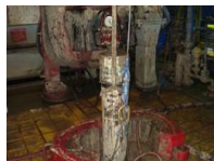
Fig. 2 – Tie onto the casing
