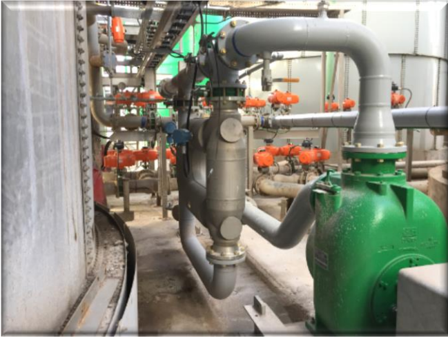
Figure 4 – In-line Coriolis meter (flow rates & density)
