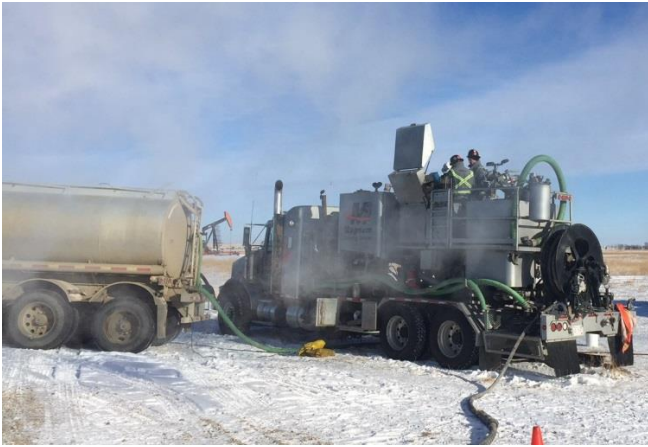
Figure 4b: preparation of expandable sealant
