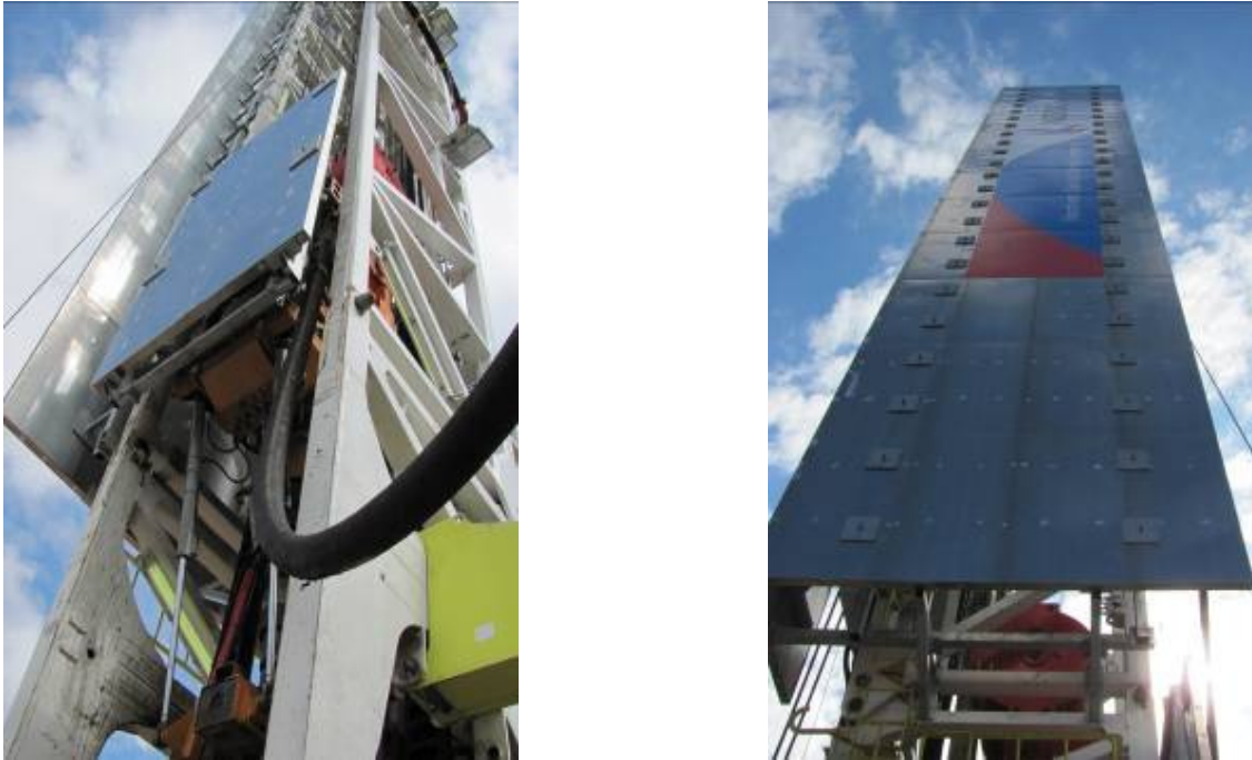
Figure 9: Sound protection on the rig.
