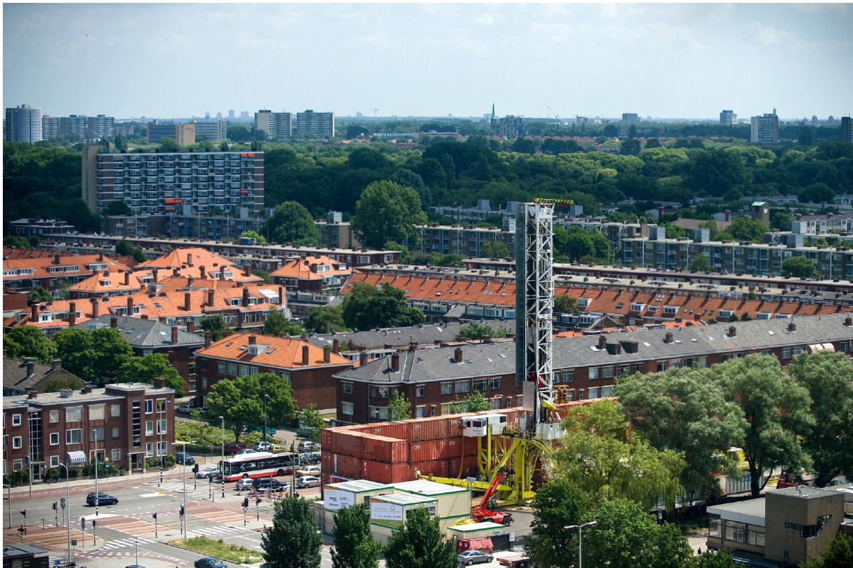
Figure 10: Drilling in a densely populated location with minimal impact.
