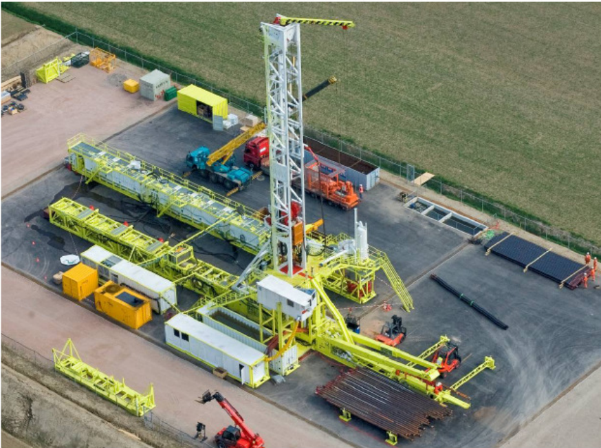
Figure 1: LOC 400 drilling rig on location in the Netherlands
