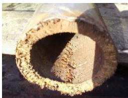
fig 5 Typical jet cut
