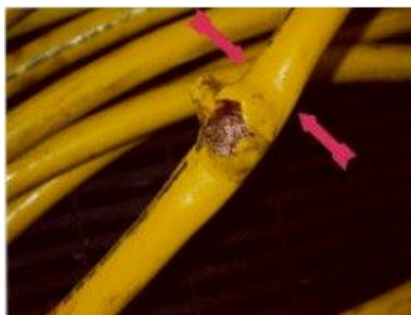
Fig. 14 - Parker hose ruptured.
