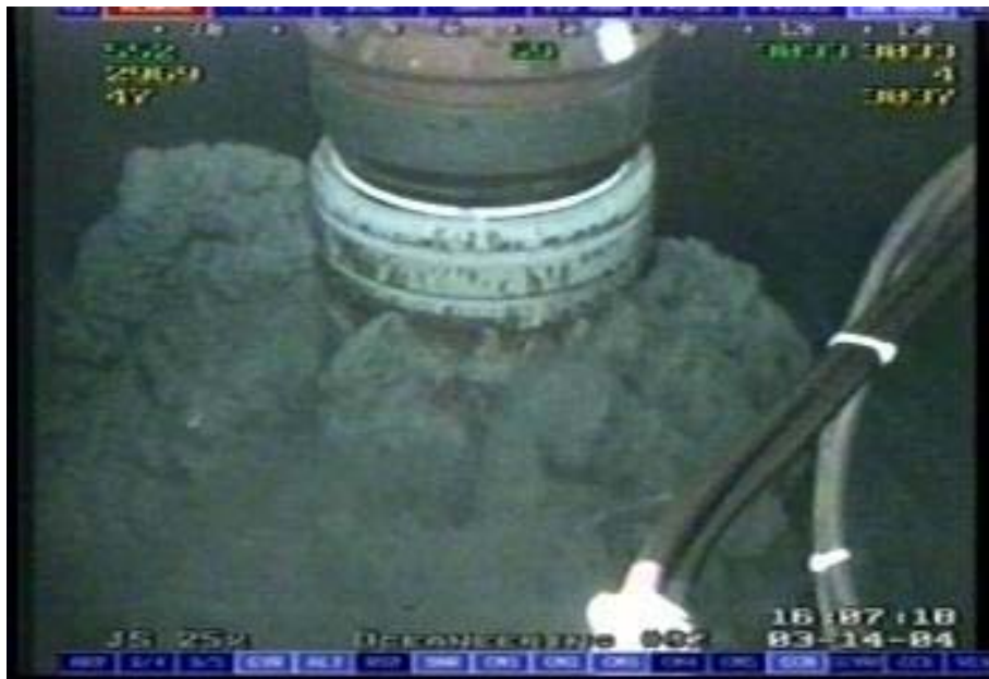
Fig. 9—Cement returns at the seafloor on a 22-in. riserless job.
