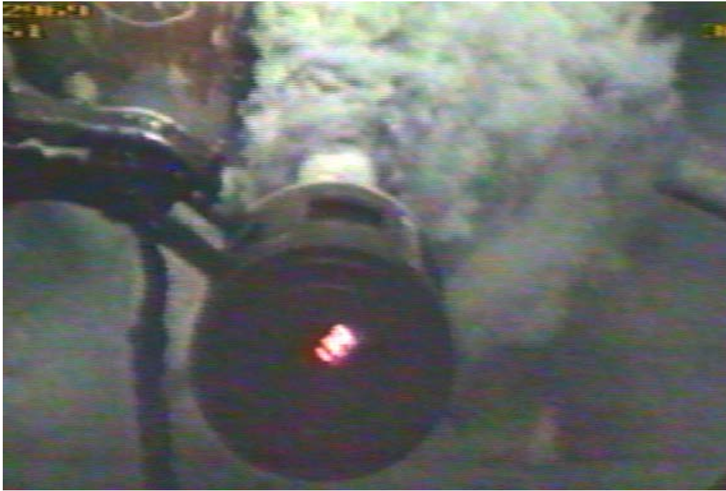
Fig. 12—Foam cement returns identified using pH meter reading 13.6.
