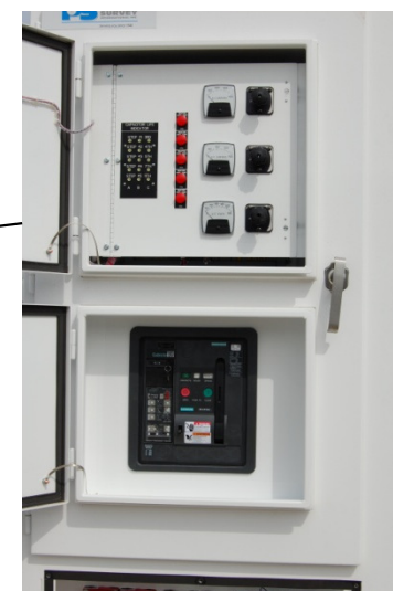
Main 600 V Electric Disconnect (behind panel) door
