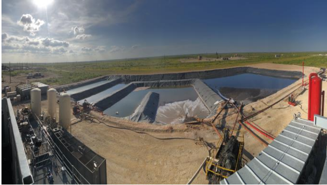
Figure 1 – Water Storage Pits
