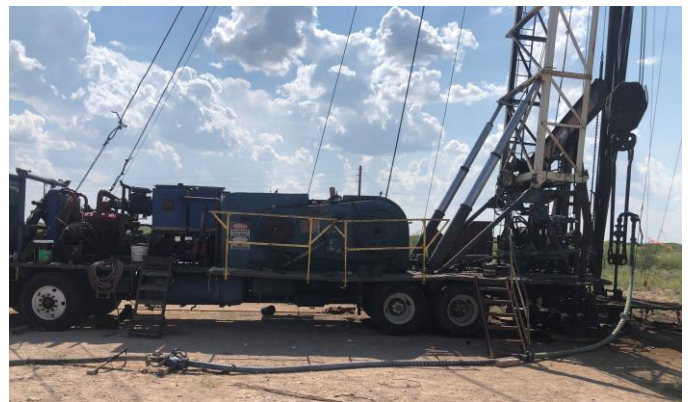
Fig. 3: placement of AAM material
