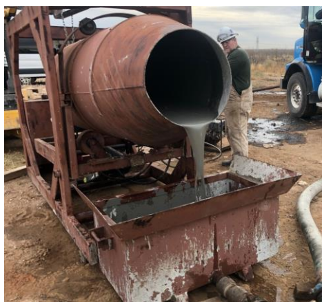
Fig. 6: preparation of slurry for pumping
