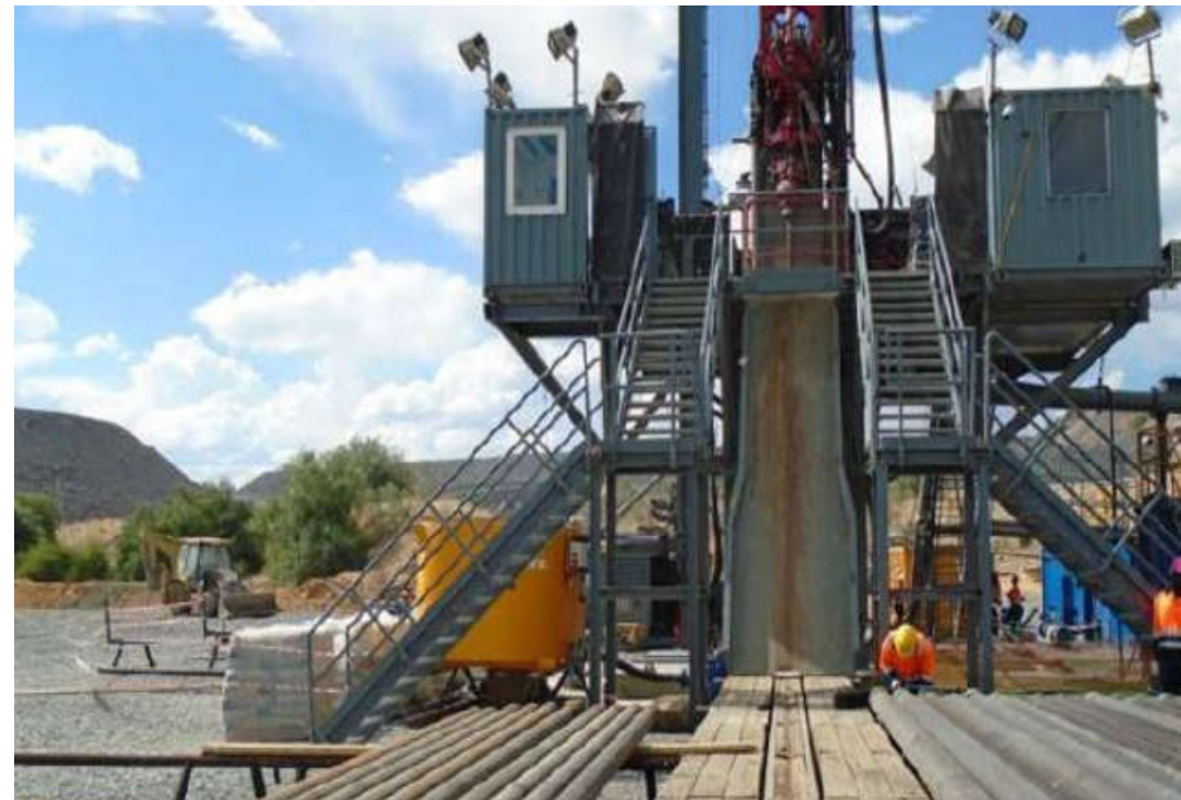
Rig for Coring Application in Diamond Mine
