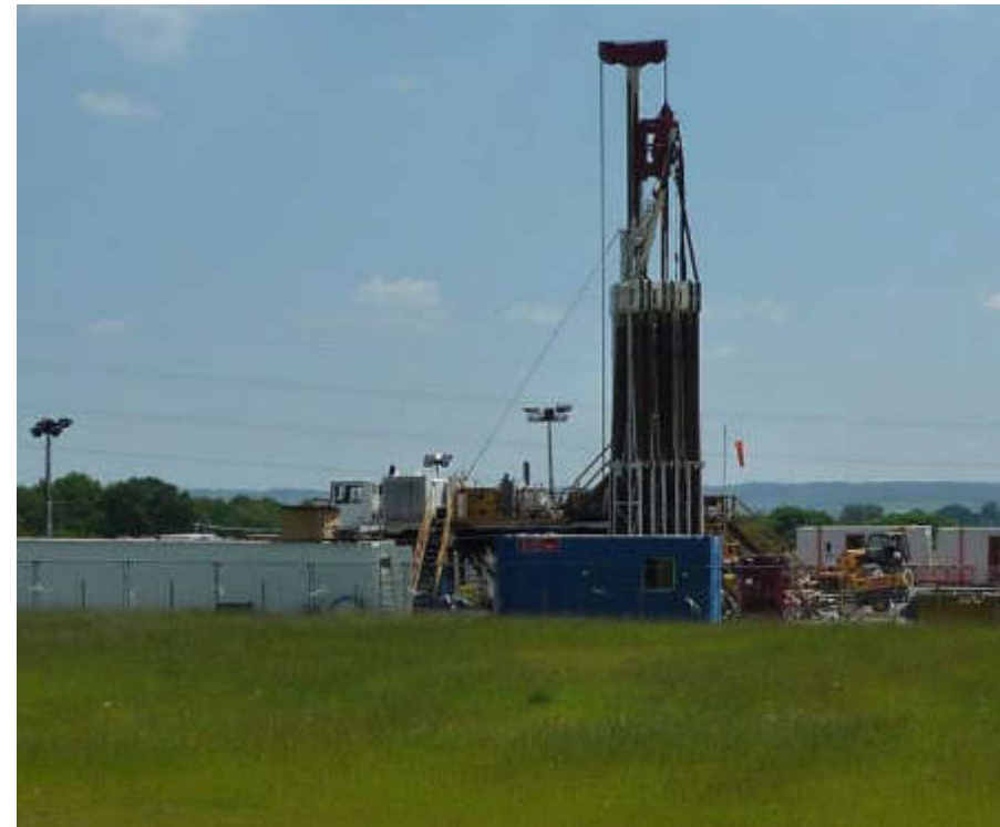
Geometric Drilling Rig HH55
