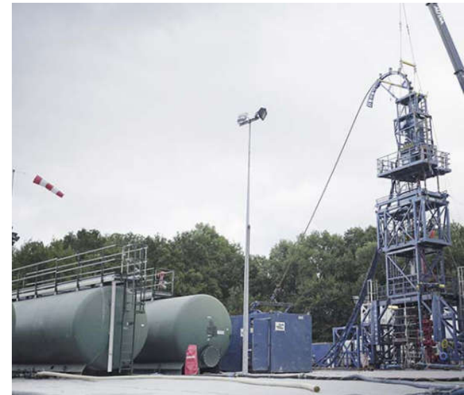
Coil Tubing Casing Exit Operations- Courtesy of
