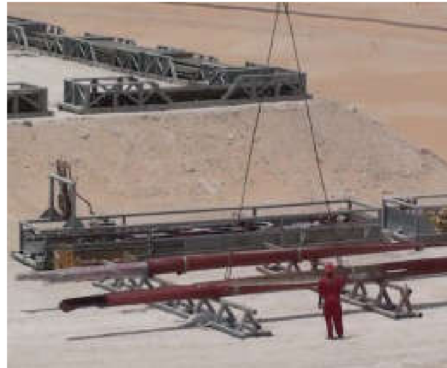
Lifting operation of 18-5/8-in system
